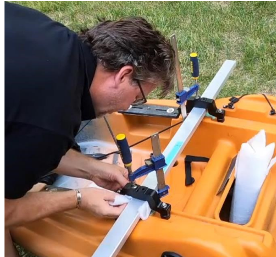
Packing foam works to temporarily stabilize joint during upcoming drilling procedure.
